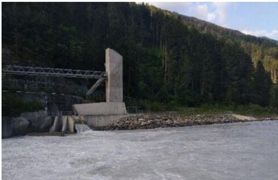
Figure 80: Fish lift Runserau, Austria (source: M. Schletterer)
