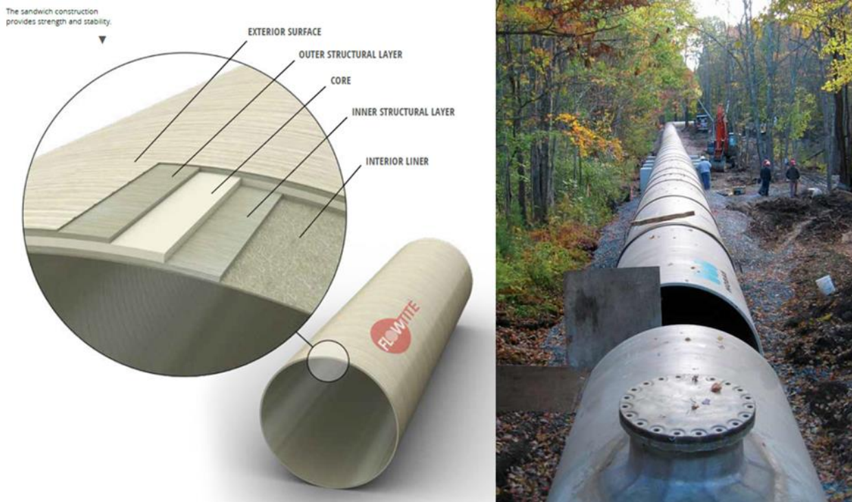
Figure 73: Flowtite pipe structure (left) and replacement of a wood stave penstock segment by a Hobas GRP pipeline (right). Jackman Hydro Station, Hills-borough, New Hampshire, USA (Amiblu, 2020)
