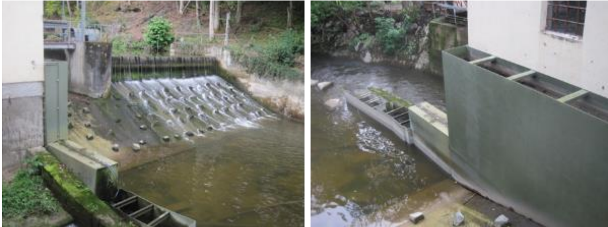
Figure 81: Fish lock at the Jeging 2 HPP, Austria. (source: M. Schletterer)
