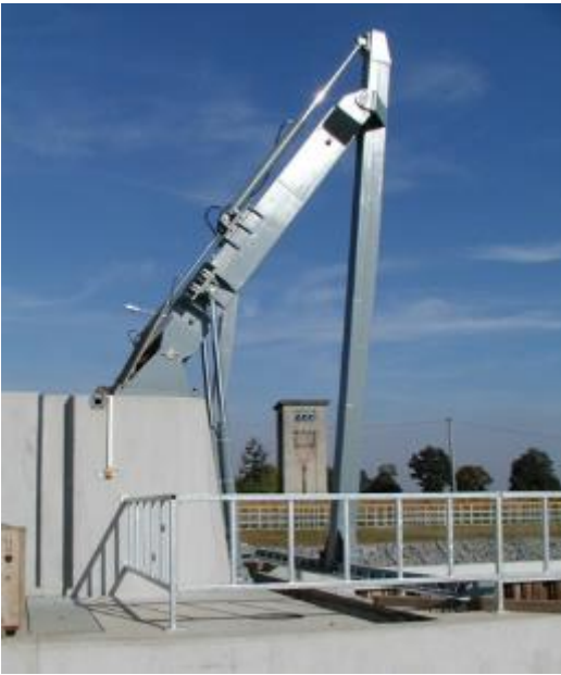
Figure 59: Articulated trash rack cleaner in Januszkowice SHP - Oder river, Poland (source: J. Steller)
