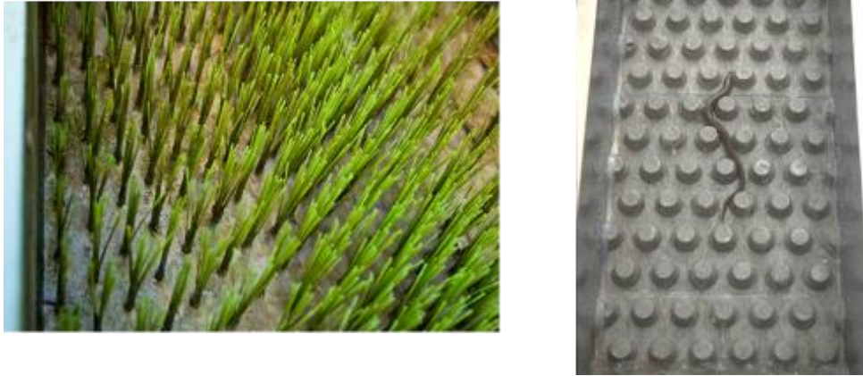
Figure 79: Eel ramp covered by a brush type substrate (left) and (right) a concrete cones substrate (source: AFB)
