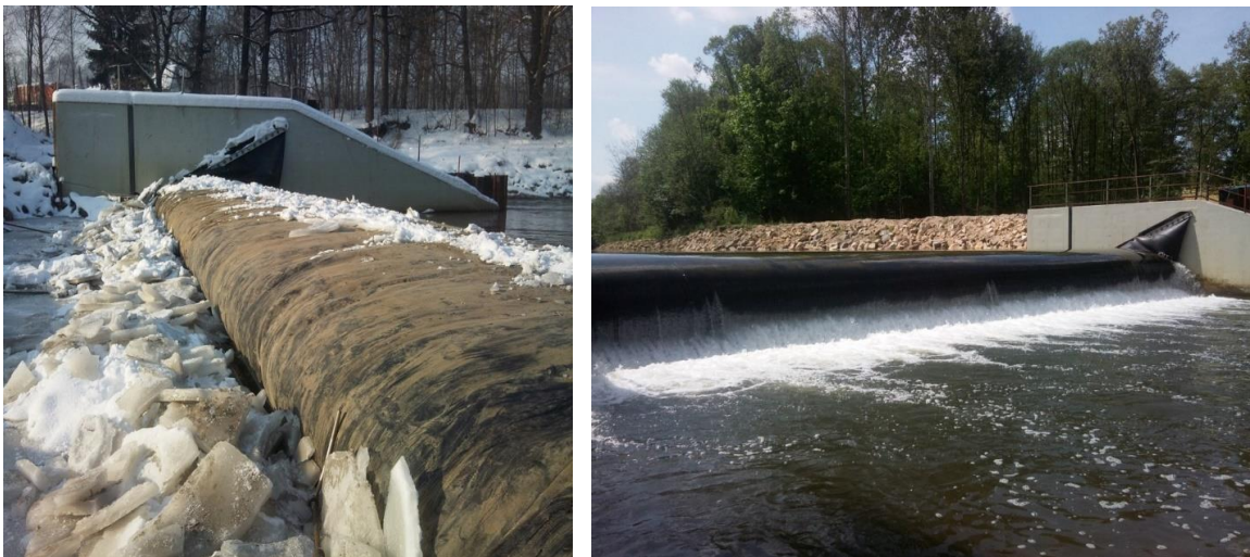
Figure 67: Inflatable weir in winter and summer seasons, Kliczkow SHP - Kwisa river, Poland (Polniak, 2015)
