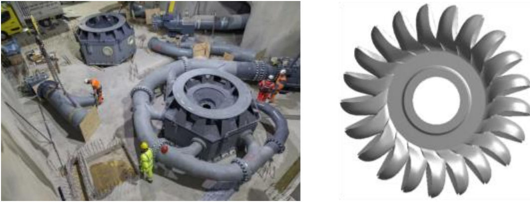
Figure 16: The 7 MW Pelton turbine of Gletsch Oberwald (CH) Hydropower plant (source: FMV SA)
