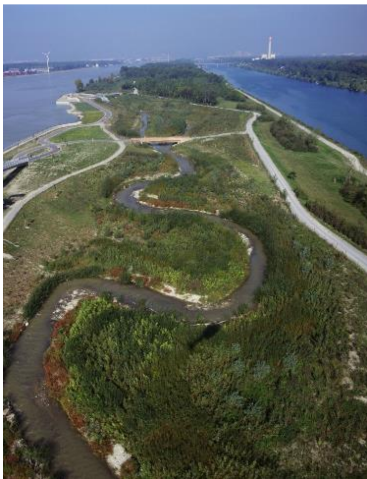
Figure 78: Nature like fishway at Freudenu HPP, Austria (source: W. Reckendorfer)
