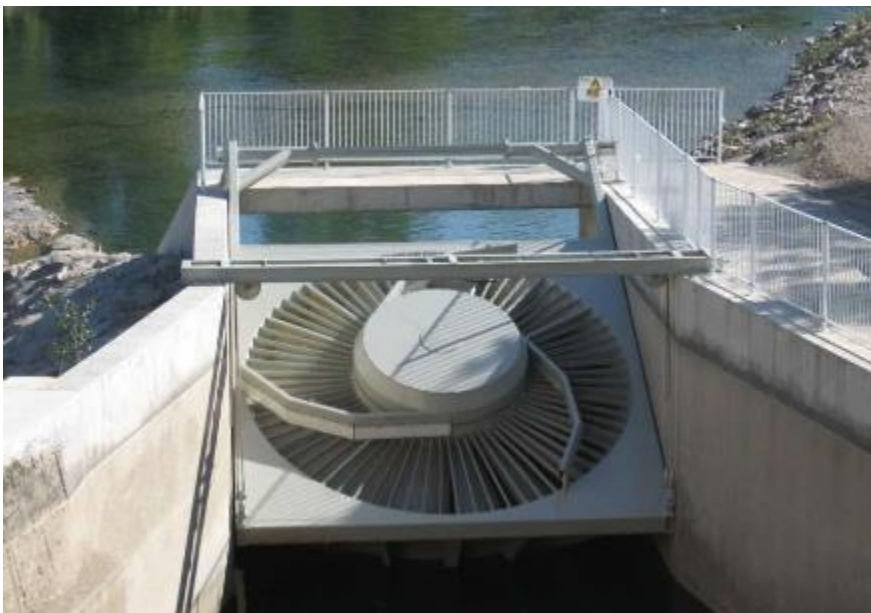
Figure 32: A VLHT unit at outlet of the Milleau canal (Leclerc, 2008)
