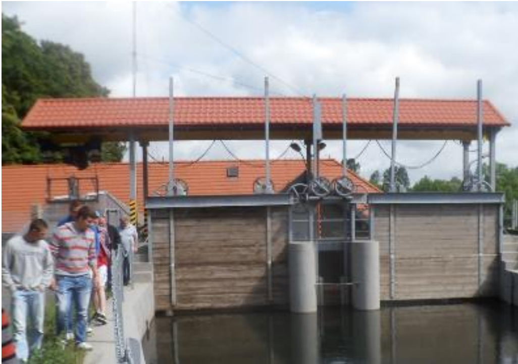
Figure 61: The Rutki SHP water intake - Radunia Cascade, Poland (source IMP PAN archives)
