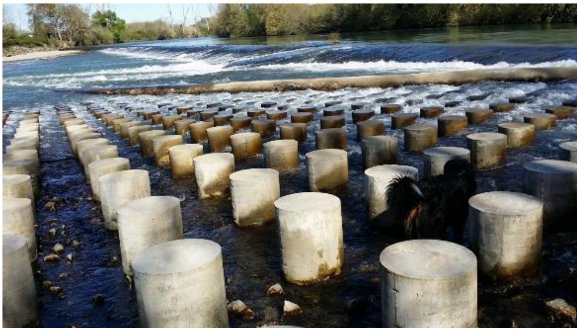
Figure 77: Combination of different types of ramps, with concrete elements in the foreground and steep, rough ramp in the background (source: P. Rutschmann)
