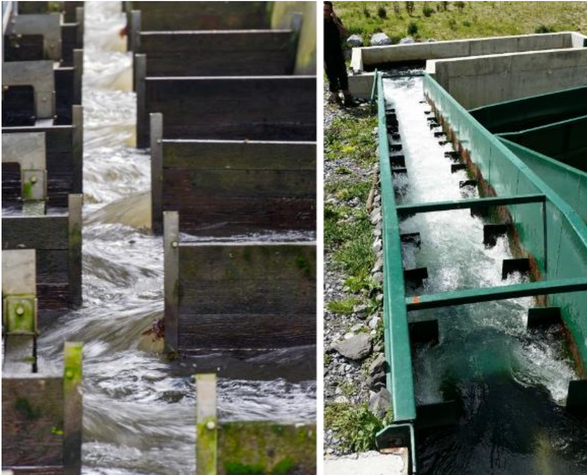
Figure 76: Pool type (left) and steep baffle type (Denil) fish pass (right) (source: J. Geist, P. Rutschmann)
