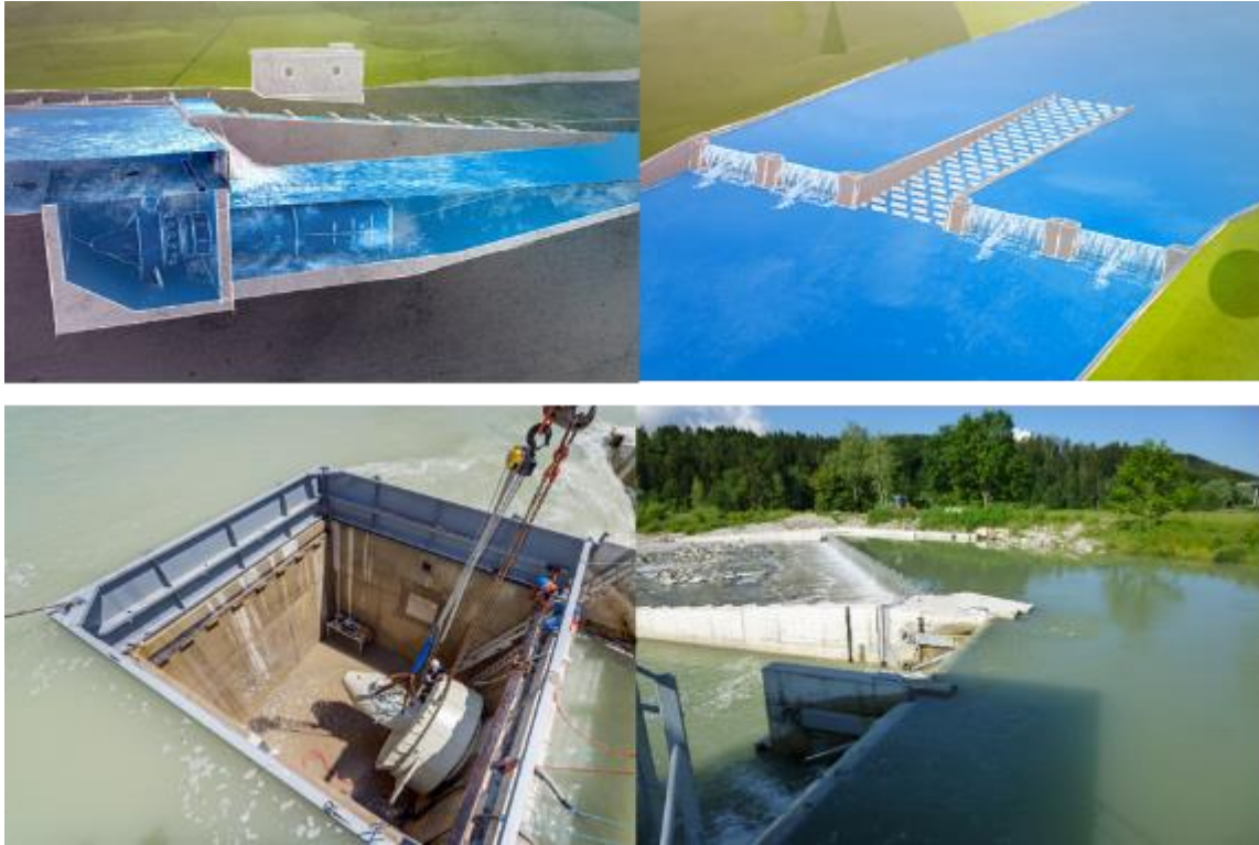
Figure 92: Visualization of the Hydro Shaft Concept (top line) and 450 kW at Grossweil, Germany (bottom line) (Source: top line: TUM and bottom line: A. Sepp)
